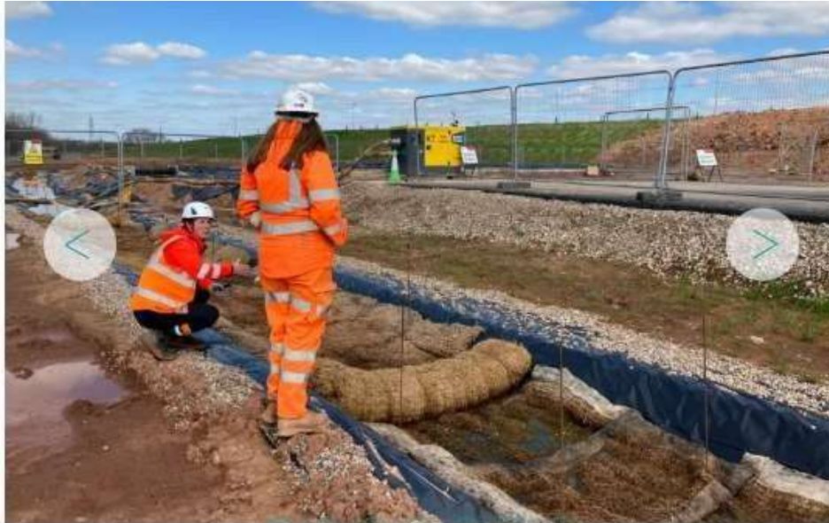
Plate 5 Silt Matting used on construction sites to capture silt or suspended solids
