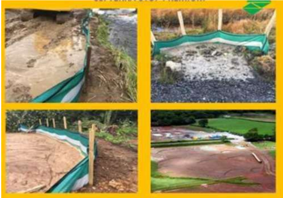
Plate 9 Silt fencing.
